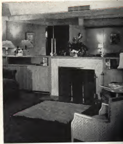
3. Cool Air Intakes In Corners of Rooms. (Ducts between Walls). Warm Air Outlet Below Ceiling.
